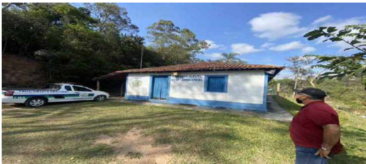
VISTA BASE GUARDA CIVIL AMBIENTAL
